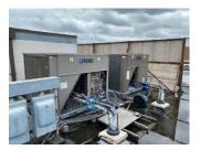
This individual air-handling unit is constant volume with the same inadequacies as previously described. Tempered air is ducted from the air-handling unit to the diffusers in the light fixtures. There are (22) additional electric resistance re-heat coils thought the ducted area. Return air is provided through the plenum ceiling.
